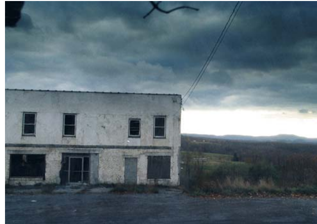
At a curve overlooking the Sewell Plateau stands the dilapidated, abandoned Lee's Tree Tavern, a two-story cinder block structure, intruding on the Trail's natural beauty.
